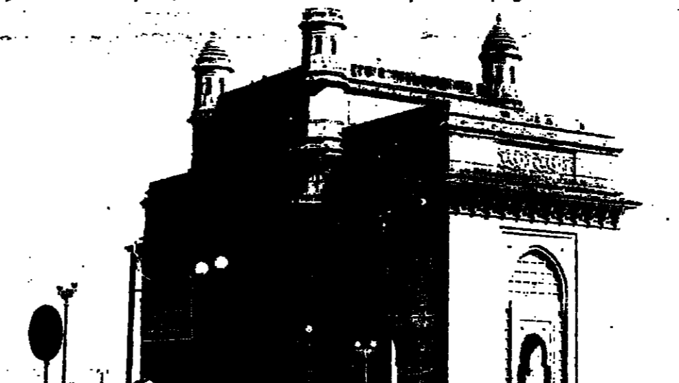
GATEWAY: The Gateway of India, which was built in 1911 to commemorate the landing of George V and Queen Mary in Bombay. It is one of the tourists' attractions in the city.
